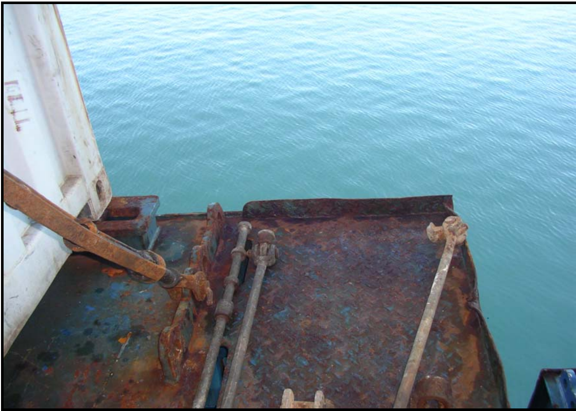
Photo 1 – Lashing Platform From Which Stevedore 1 Fell
