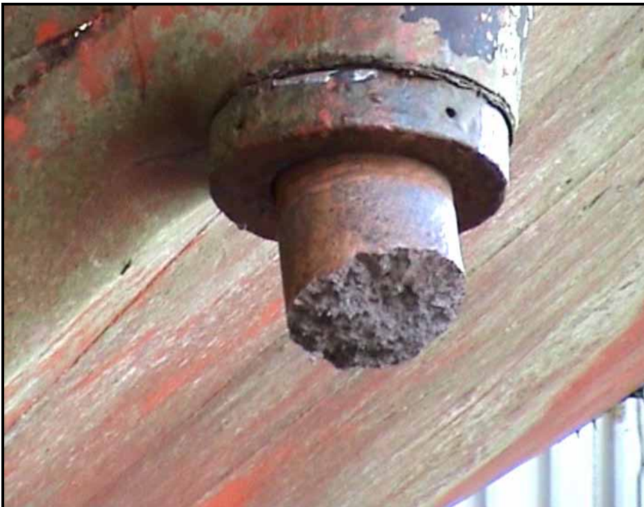
Photograph 6 Rudder. The rudderstock has been sheared off with a cant to port indicating a blow from the starboard side.
