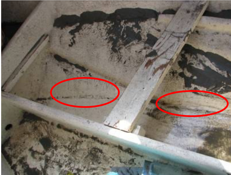
Figure 10 Fractures in the fibreglass floor beneath a seating squab
