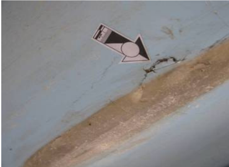
Figure 6 Impact damage on the keel
