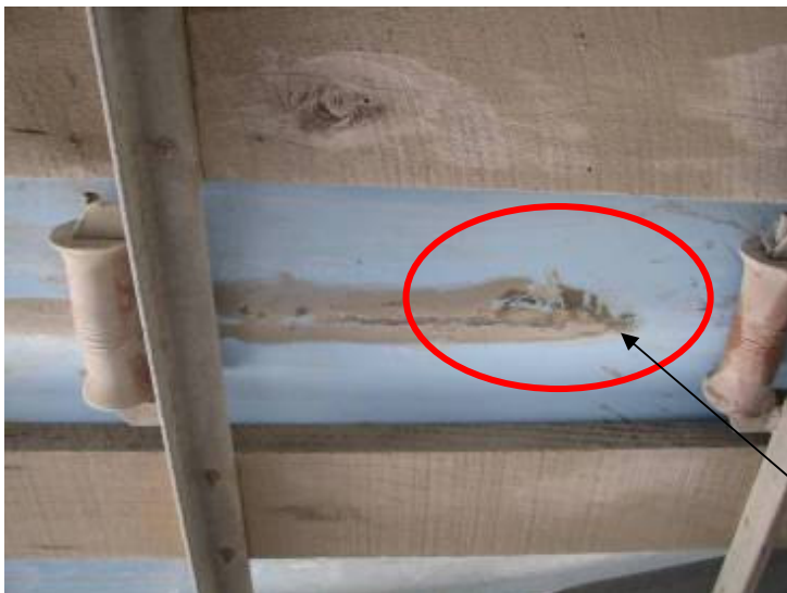
Figure 4 The 115mm jagged crack in the keel, midships
