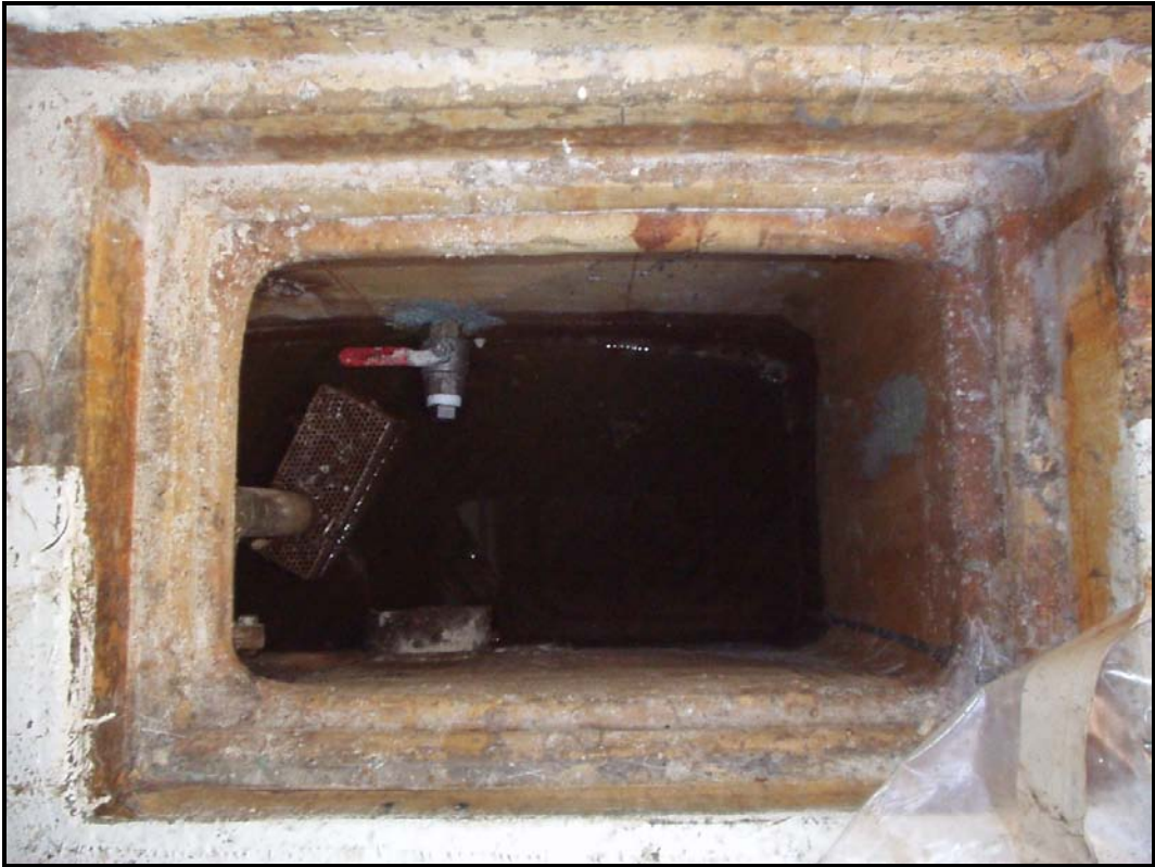
Photograph 3 Starboard Bilge Sump
