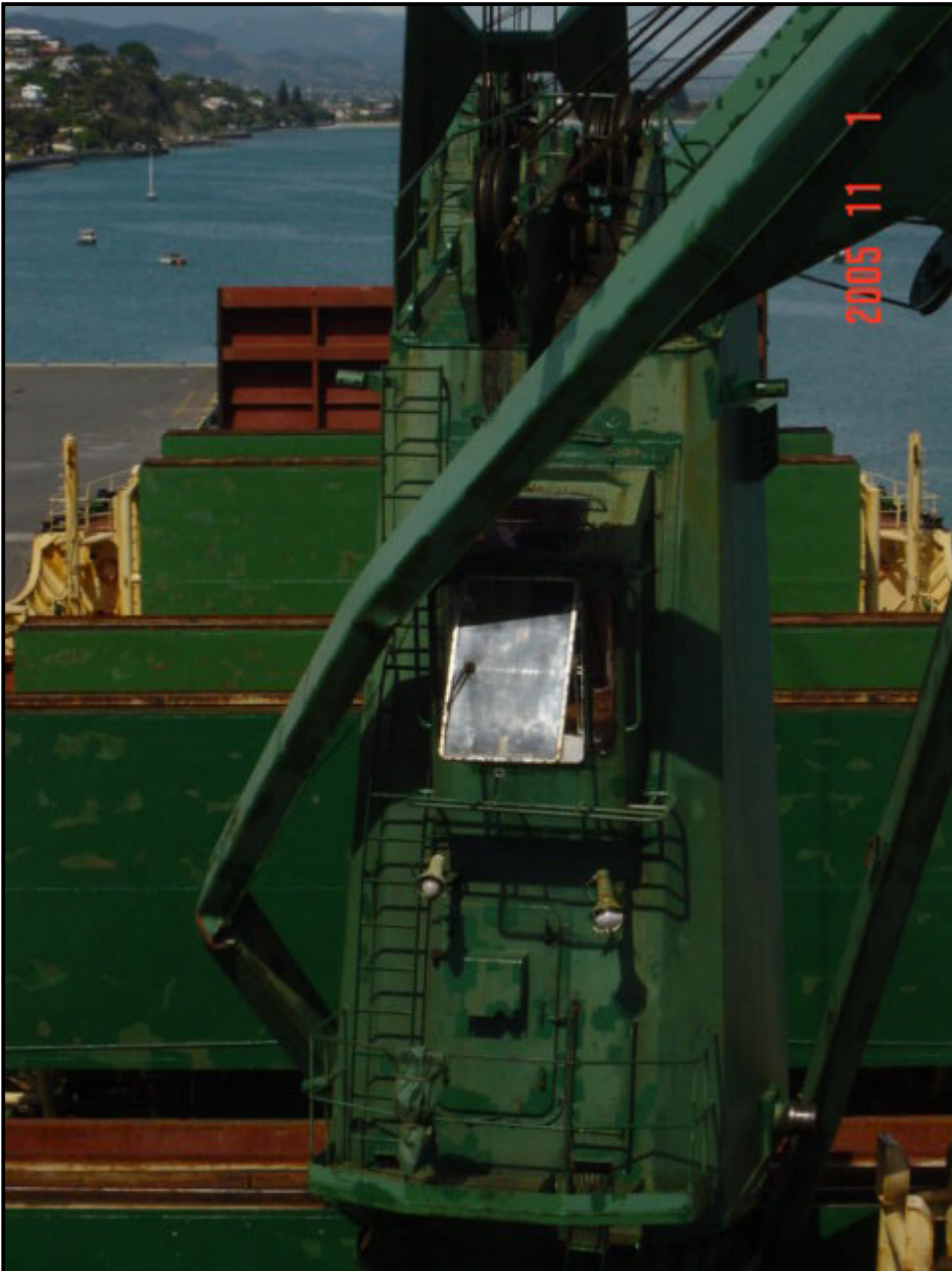
Photograph 2 Photo showing damaged No. 3 crane jib.
