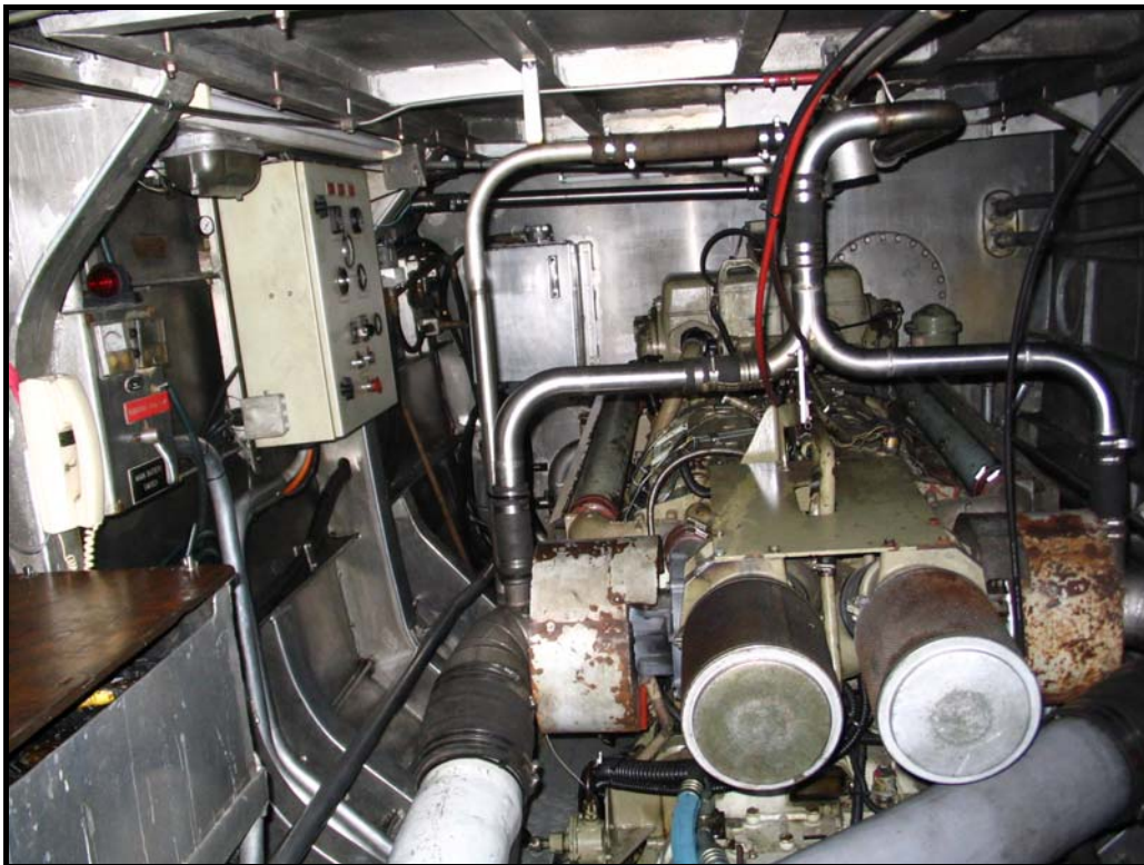
Figure 6 - View of Starboard Engine Room From Aft
