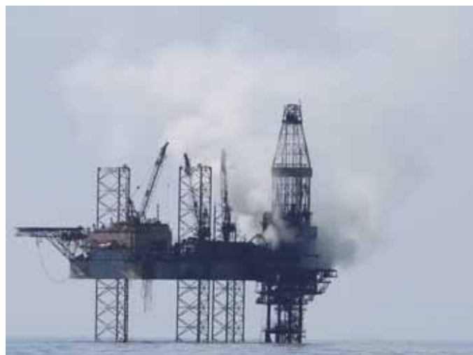
Montara well head platform
