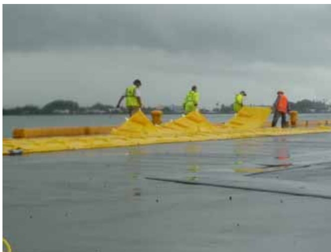
Boom laid out in readiness for booming around the vessel
